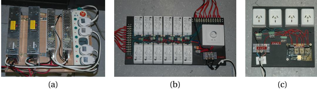
Figure 31: Power Supply. (a) TEC cooling supply (b) Halogen Illumination supply. (c) Controlled Illumination relay.
